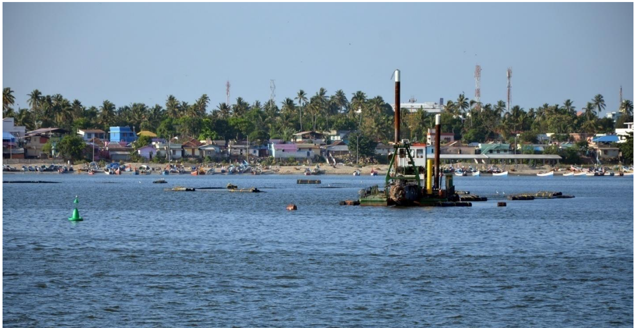
Fig.4 Construction Site inside the Kollam Port
